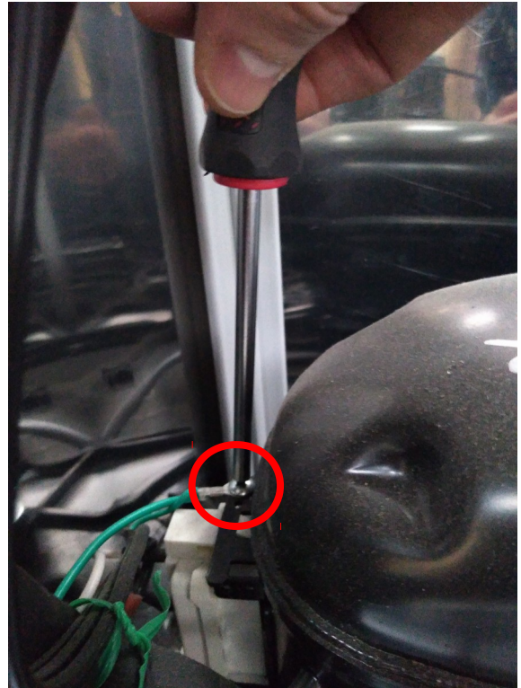
10- With a #2 Robertson screwdriver screw the ground eyelet (green wire) in the compressor bracket.
